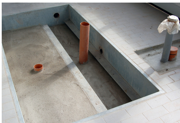
Fig. 1: Assembling case concret-casted (example)
