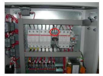
Caution: check that the pump is correctly connected and functioning (on first start-up only). To do this turn on the machine and listen carefully to hear the liquid hitting the blades of the rotor. If you cannot hear this noise despite hearing that the pump is functioning, the power supply phases of the current need to be inverted.
