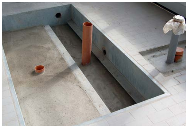
Fig. 1: Assembling case concret-casted (example)
